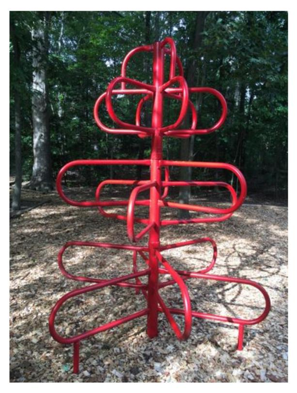
The jungle gym is in good condition, but needs repainting soon, yet it is in better condition than the swing set. The jungle gym was most recently repainted as part of an Boy Scout eagle project in 2012. Repainting in 2017 is recommended. The
