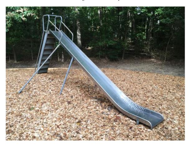
The slide has received very little maintenance over the nearly 30 years it has been in service. The site inspection found the slide to be structurally sound. There is a little rust on the upper supporting poles and under the top of the ladder, but this is a minor given the age of the slide. Some paint could be applied to cover the rust, but this is not really necessary. The slide should have an additional lifetime of at least 35 years.
