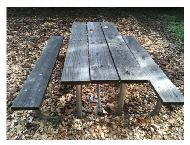
Component #7, Tot Lot Bench. A heavy-duty, 6 foot long bench was installed by the developer, Richmarr Corporation, with the rest of the tot lot equipment in the 1982-1983 timeframe. The bench is permanently mounted in the ground. It is composed of two metal tubes that support a board on the seat and another board on the back of the bench. The following is a picture of the bench.
